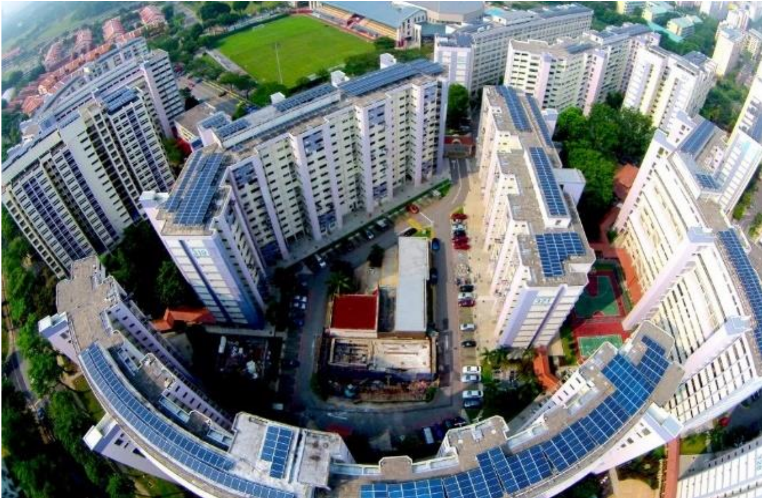
Solar Panels on Residential Buildings
