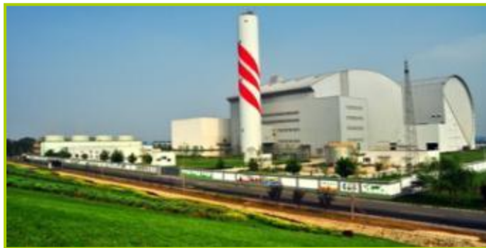
焚烧厂 Incineration Plant
