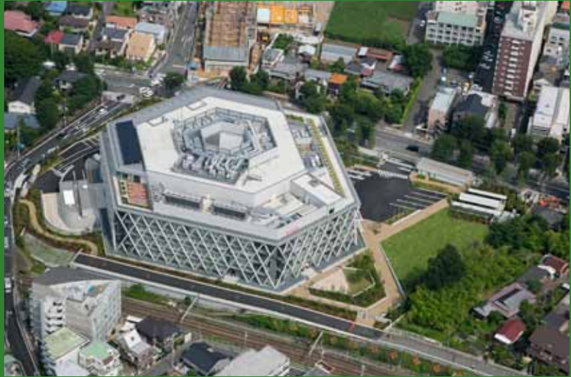
Top view of Sengawa Kewport (seen from above from the southeast)
