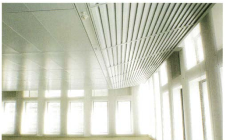
Radiant ceiling panels
